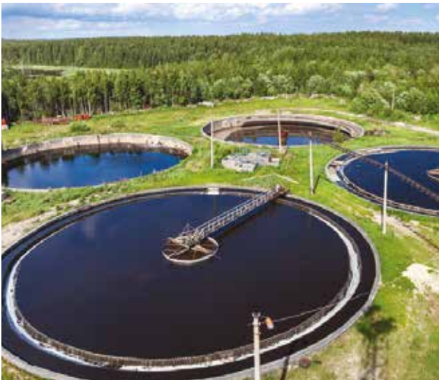
CIVIL AND INDUSTRIAL WASTEWATER TREATMENT
