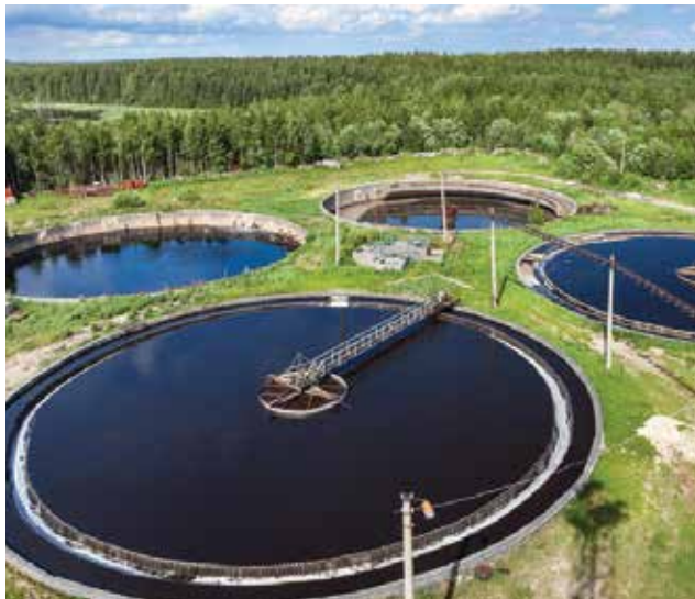
CIVIL AND INDUSTRIAL WASTEWATER TREATMENT
